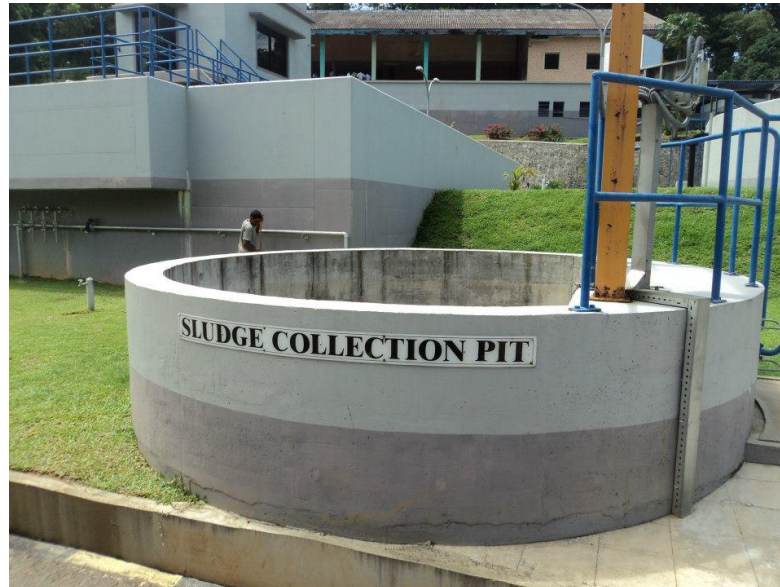
Figure 7 Sludge collection pit
