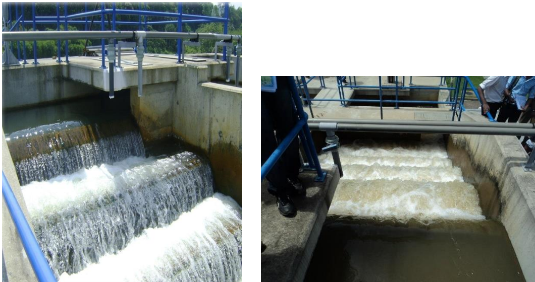
Figure 4 Cascade aerator
