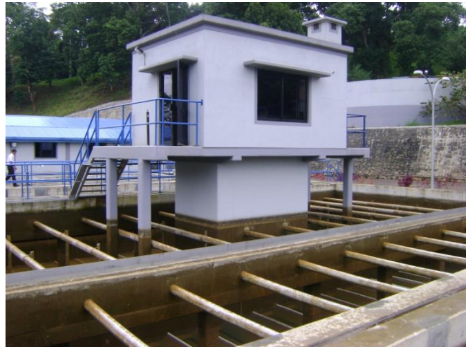
Figure 5 Pulsator clarifier
