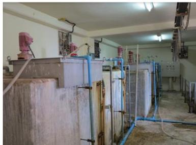
**Figure 2 Alum Solution Tank**
