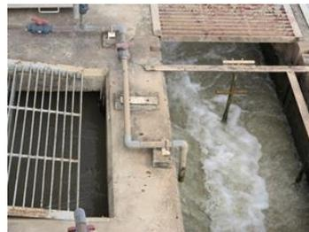
**Figure 5 Polymer injection site**
