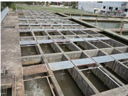
**Figure 7 Vertical Baffle Channel (8 basins)**
