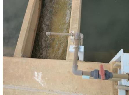
**Figure 10 Injection Line of Pre-chlorination**
