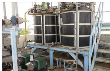
**Figure 4 Polymer Storage Tank**
