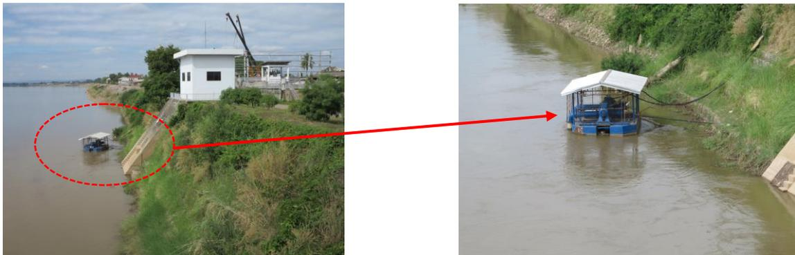
**Figure 16 Floating Water Intake Pump**
