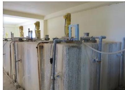
**Figure 3 Chlorine Solution Tank**
