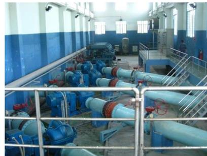
**Figure 7 Air pump system for filtration tank**
