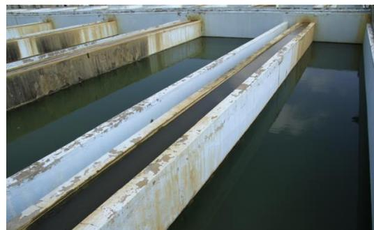
**Figure 5 Sludge Blanket Sedimentation Tank**
