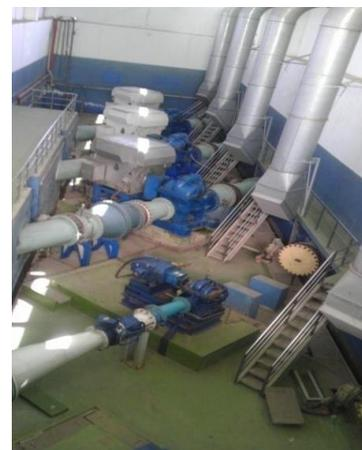
**Figure 9 Clean water pumping station**
