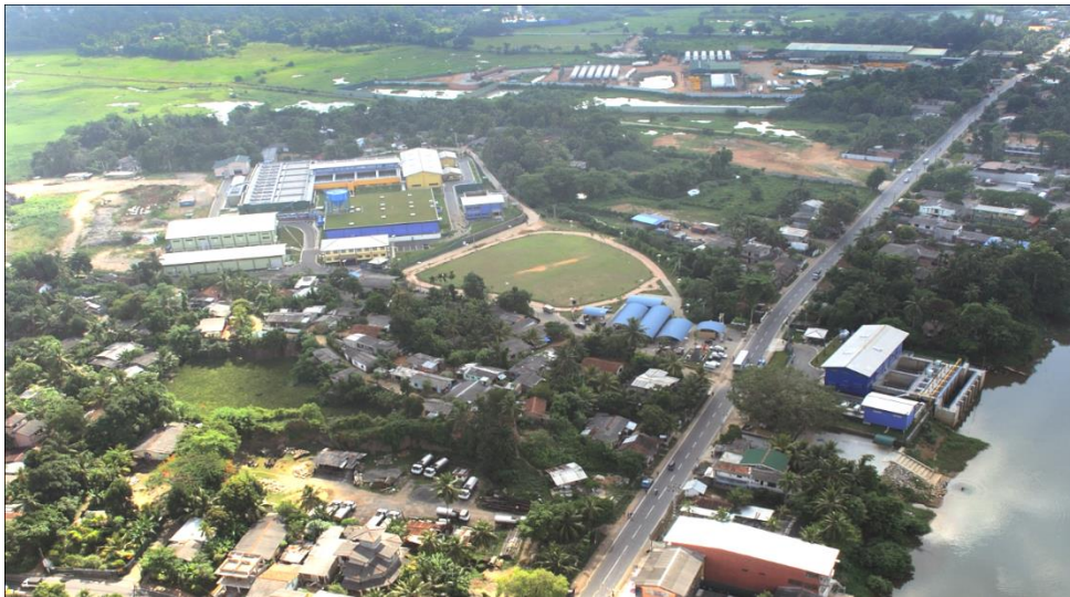
Figure 1 Biyagama Water Treatment Plant
