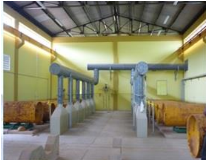
Figure 6 Chlorine Storage Building
