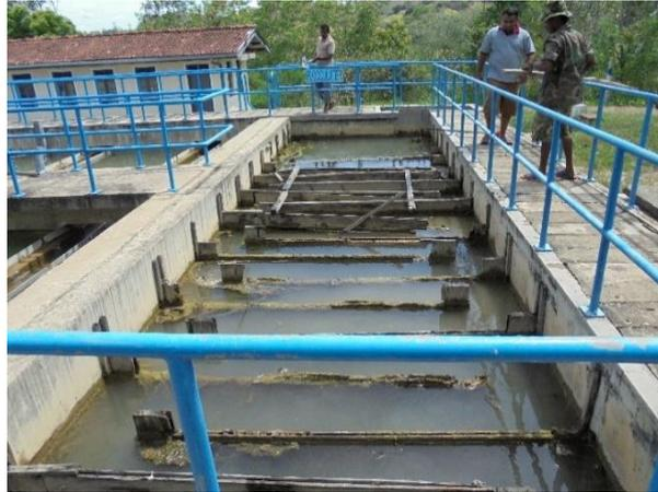
**Figure-4 Flocculation tank**
