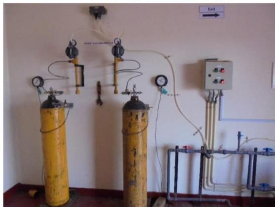
**Figure-7: Gas chlorine adding system**
