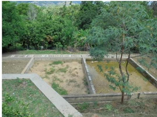
**Figure-8: Sludge drying beds**
