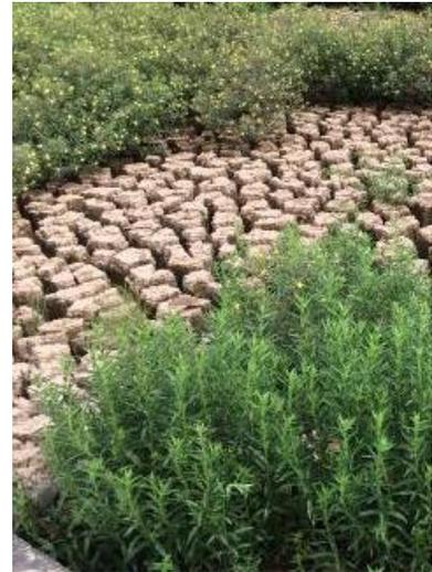
**Figure 11** Sludge drying bed
