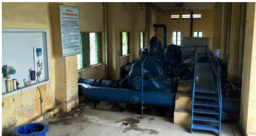
Figure 7 Pumps used in the first pumping station and backwash pumping station
