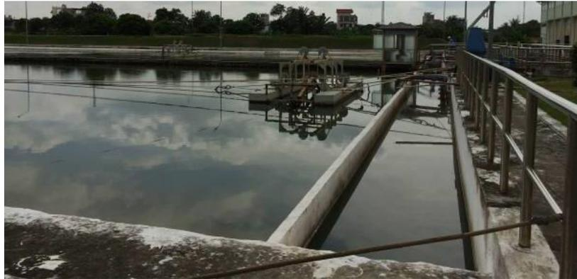
Figure 6 Horizontal sedimentation tank
