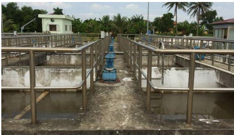
**Figure 5 Coagulation-Flocculation tank**
