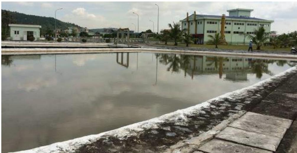
Figure 3 Pre-sedimentation tank
