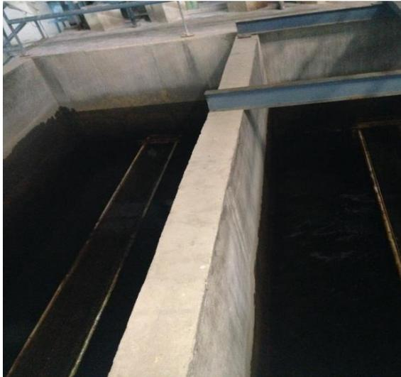
**Figure 7 Rapid sand filter**
