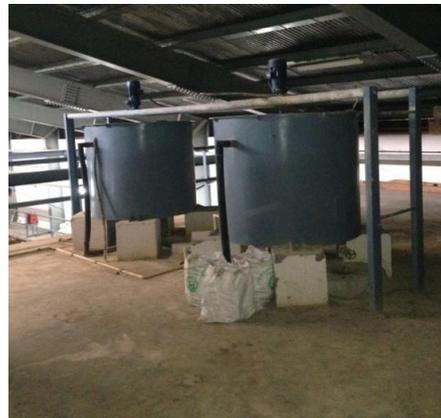
**Figure 4: Alum dosing tank with mixer**
