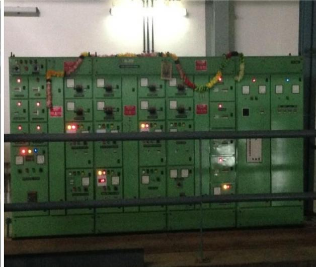
**Figure 8 Control panel for backwashing**
