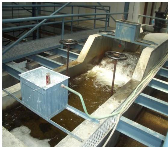
**Figure 5: Coagulation and flocculation**
