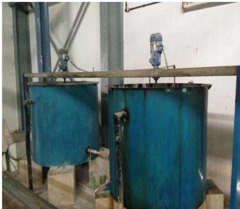
**Figure 3: Chlorine dosing tank with mixer**
