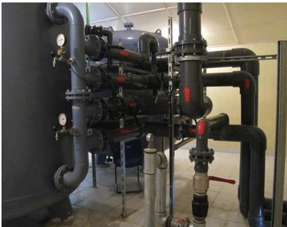
**Figure 2 Pressure filters**
