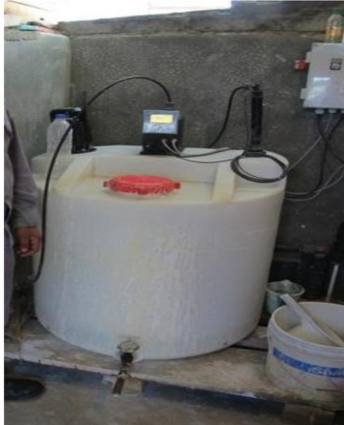
**Figure 4 Chlorine dosing equipment**
