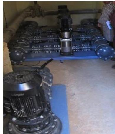
**Figure 3 Pressure filter pumps**
