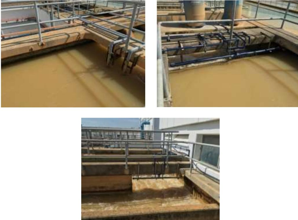
**Figure 9: Pre Chlorine, Coagulant, and Flocculants Dosing Point**
