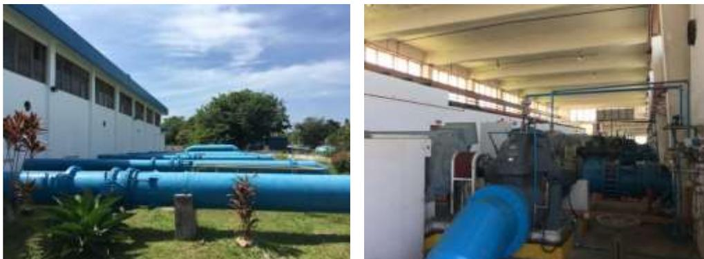
**Figure 14: High lift pump for treated water distribution**
