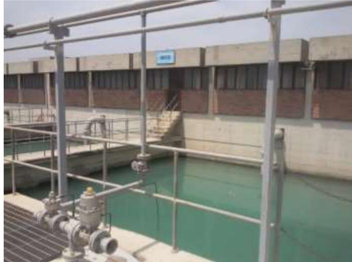
**Figure 8: Rapid sand filter**
