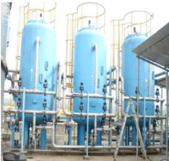
**Figure 4 Pressure filters**
