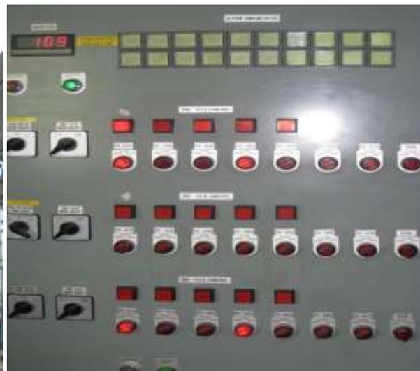
**Figure 5 Control Panel for Backwashing**
