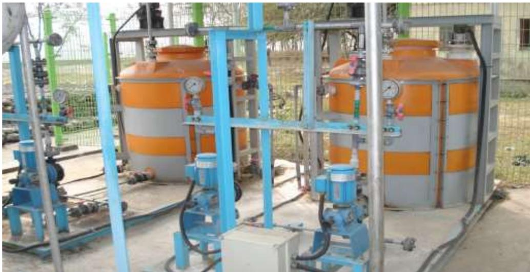
**Figure 6 Chlorine dosing equipment**
