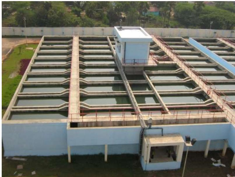
**Figure 9. Clarified water collection channels of clarifier**
