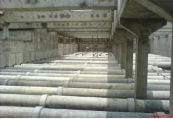
**Figure 7. Distribution pipes of Pulsator clarifier**
