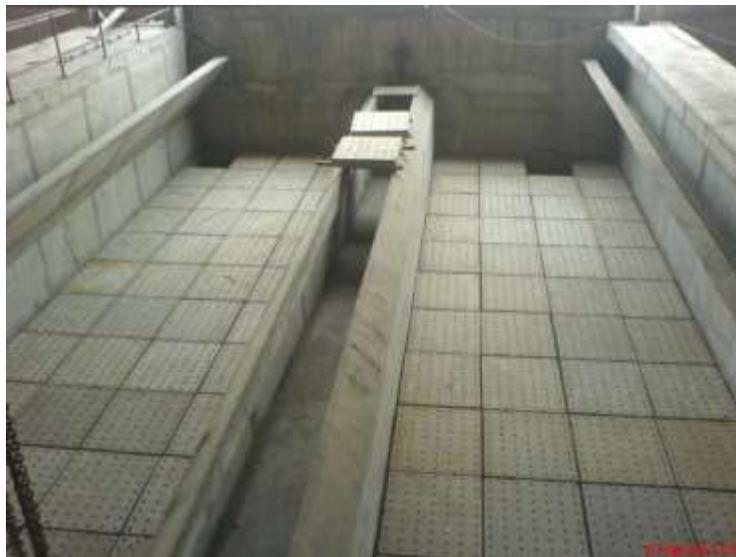
**Figure 10. Floor level of filter with perforated precast RCC slab**
