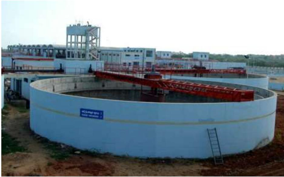
**Figure 12. Sludge Thickener**
