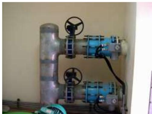
**Figure 6. Vacuum break valve**
