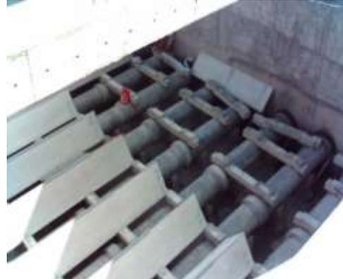
**Figure 8. Distribution pipes with deflectors of Pulsator clarifier**
