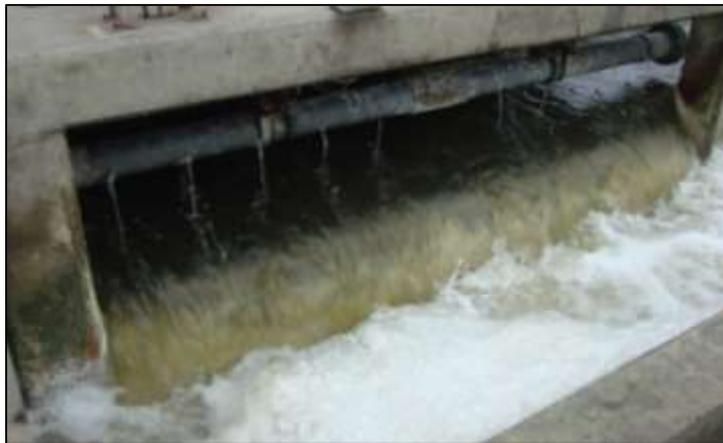
**Figure 4 Injection of Alum**
