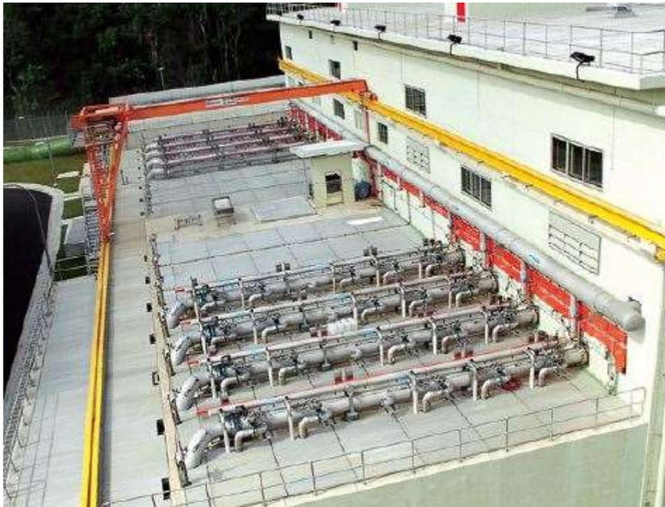
**Figure 5 Siphoning to operate the UF process**
