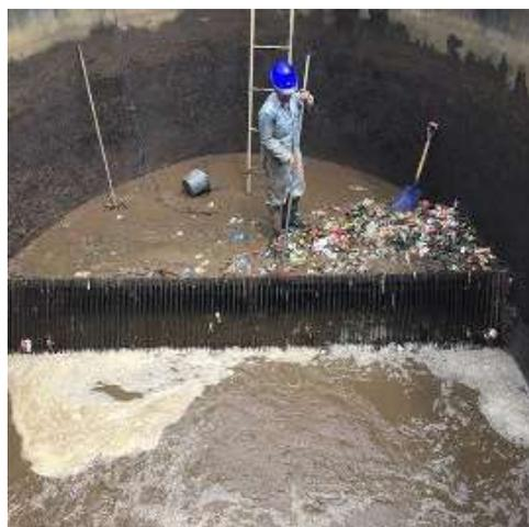
**Figure 4 Cleaning at the Cikapundung river water intake**
