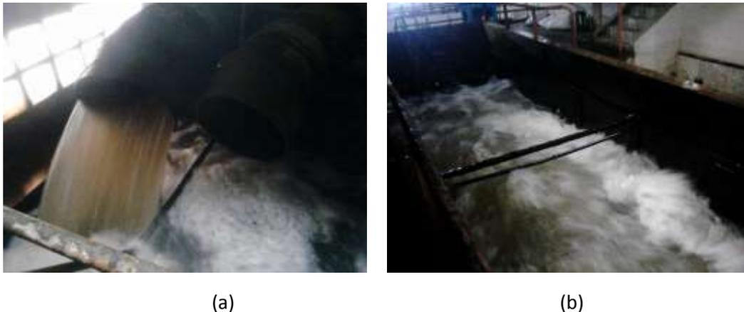
**Figure 5 (a) Collecting chamber 1 receiving water from Cikapundung river, and (b) collection chamber 2 receiving water from Cisangkuy river with bar screen**
