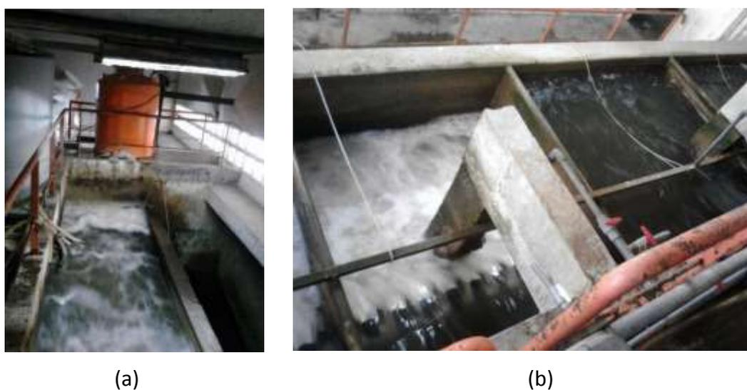
**Figure 6 (a) PAC injection point and (b) chamber to divert water to clarifier and baffle chamber**
