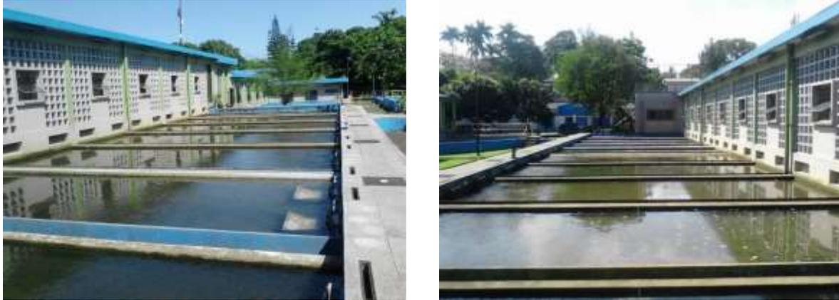
**Figure 9 Rapid sand filter unit in Badak Singa WTP**
