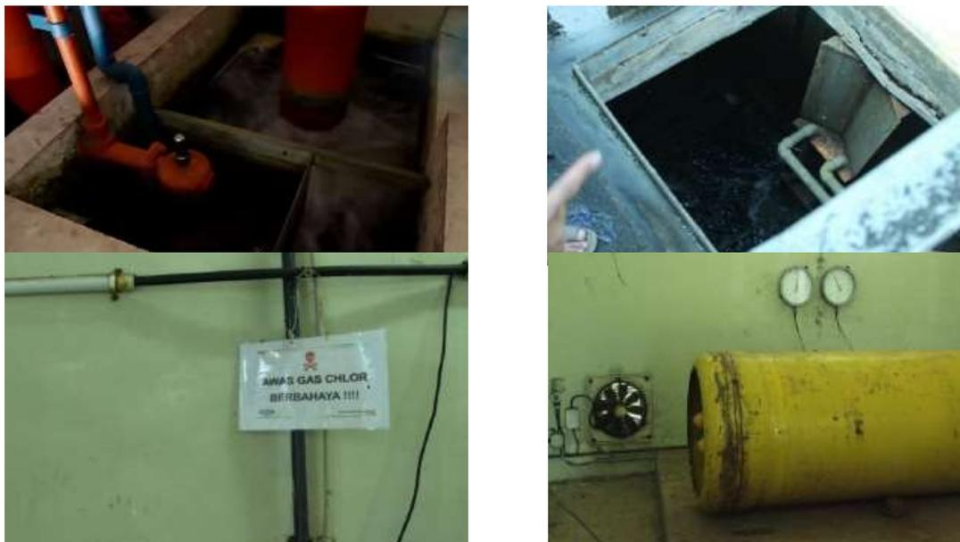
**Figure 10 Chlor injection point and chlor storage room**
