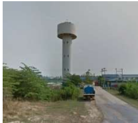
Figure 10 Elevated tank at Paisadao WTP
