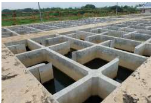
Figure 5 Baffle channel type
