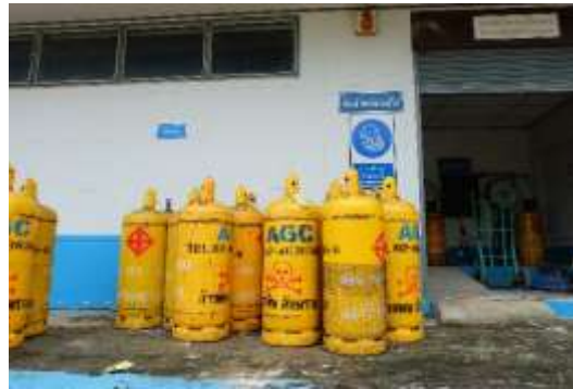
Figure 3 Chlorine containers
