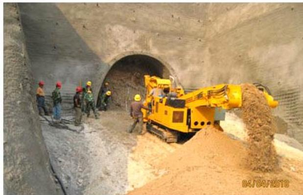
*Figure 1: Excavation of tunnel to divert raw water from Melamchi (Melamchi Water Supply Development Board, 2013)*
