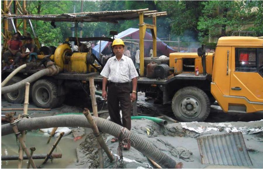
*Figure 3 Installation of production tube wells in one of the project sites (KWASA, 2011)*
