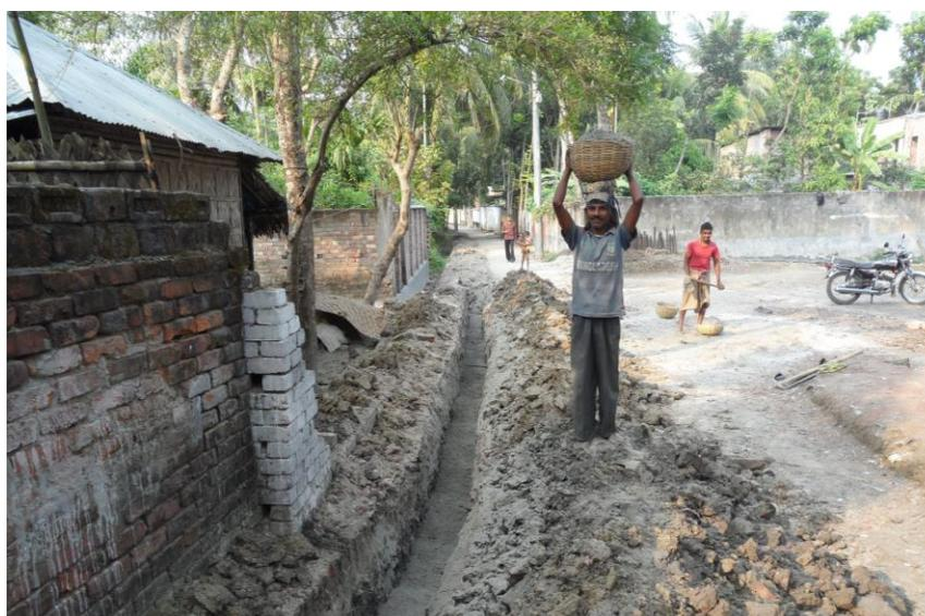
*Figure 5 Construction of trenches for KWASA's water supply network expansion (KWASA, 2016)*
