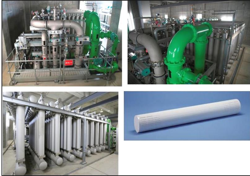
Figure 4 | Membrane filtration facility at Kawai
