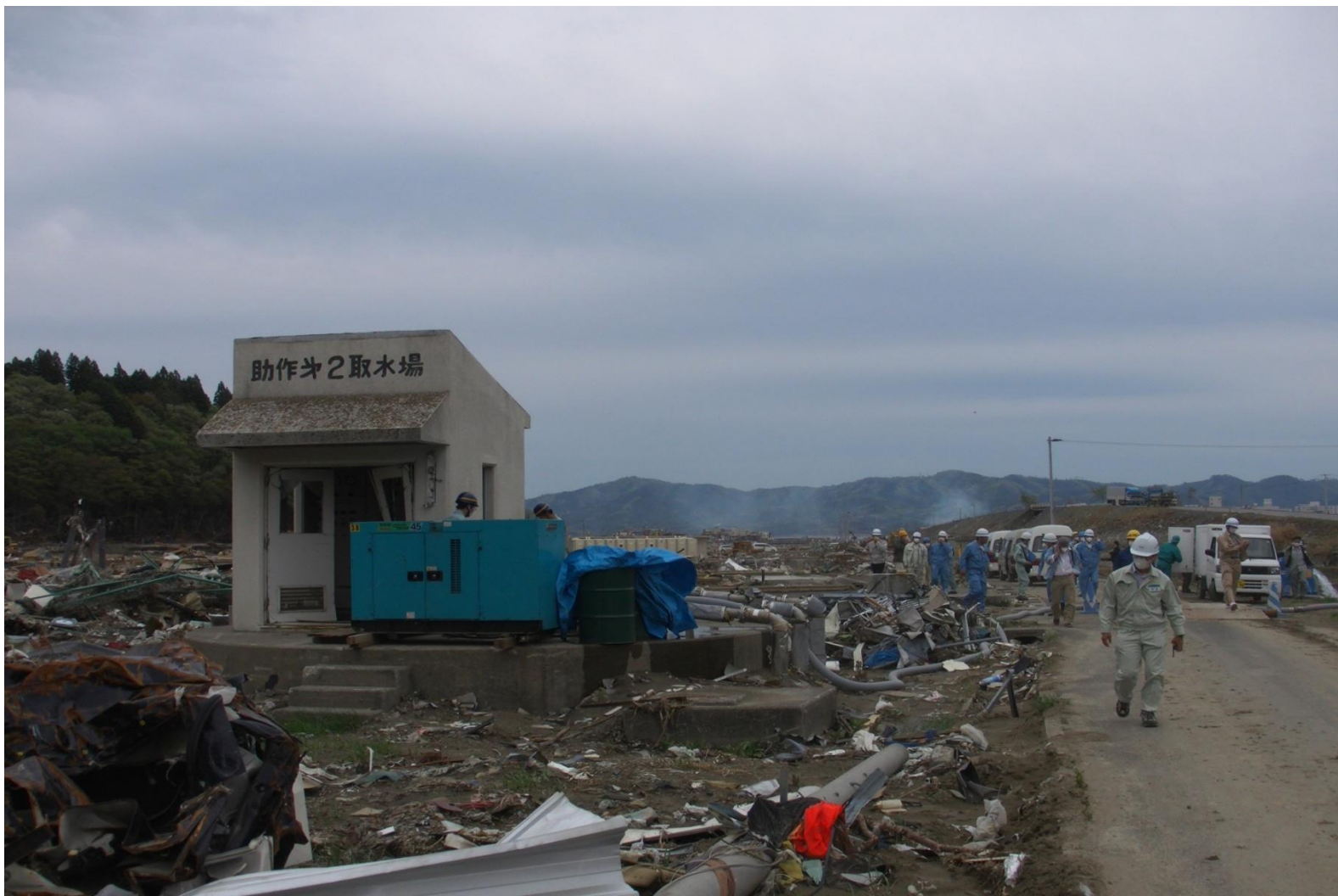
Damage to No.2 Sokedukuri Intake Facility in Minamisanriku Town
