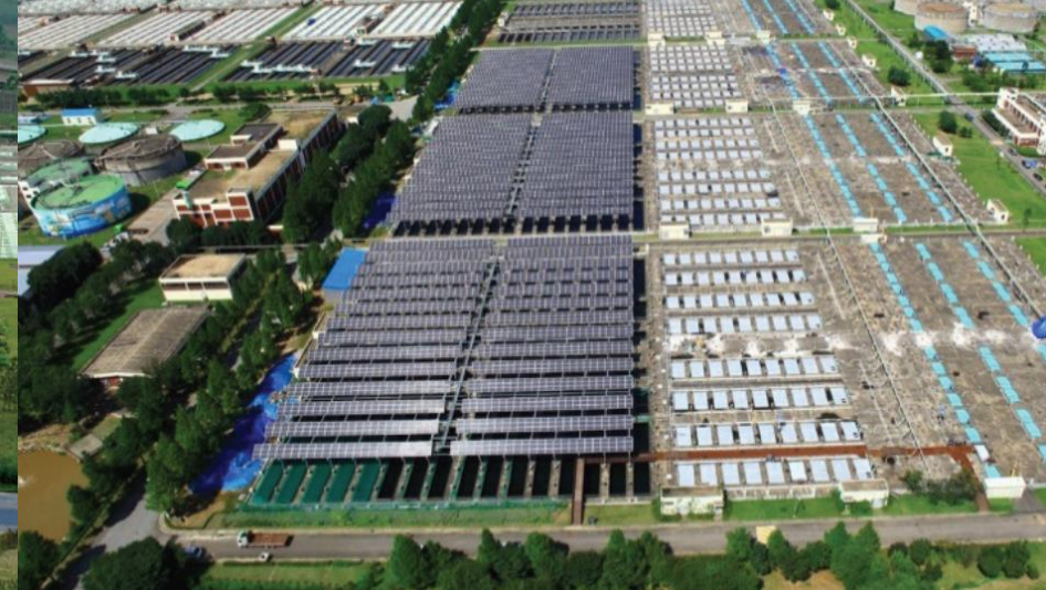
Seo Nam WWTP 1.63 M m 3 /day
