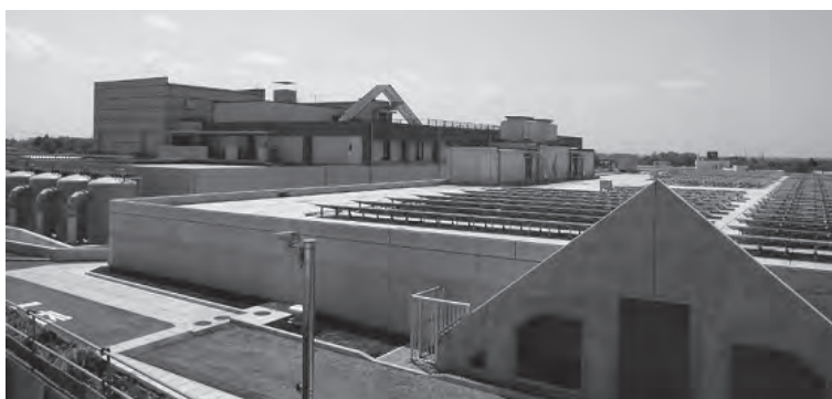
Kawai Purification Plant (CERAROCCA)
