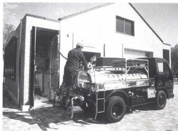
▲給水車用給水栓
