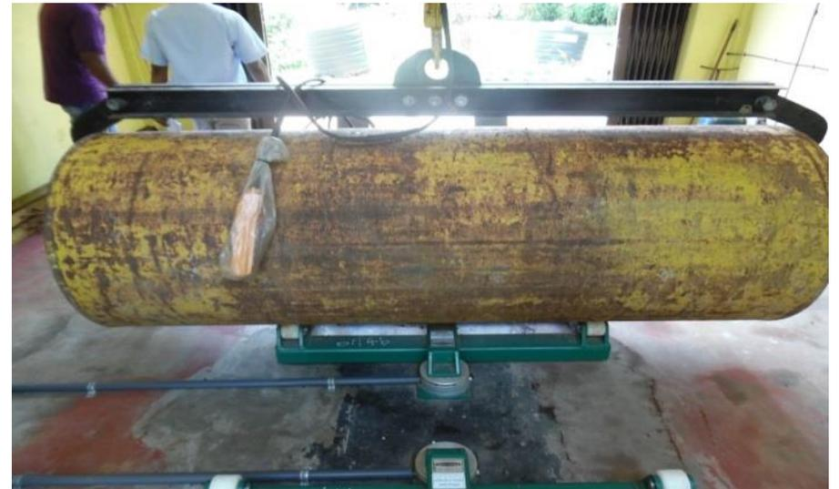
**Gas chlorine cylinder on weighing gauge**
