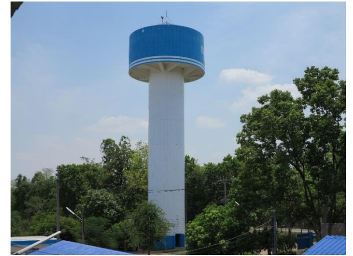
Elevated Tank for Backwashing (500 m 3 )
