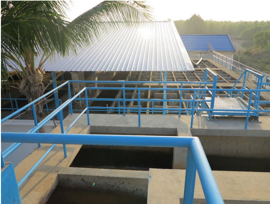
Roof of the Sedimentation Basin
