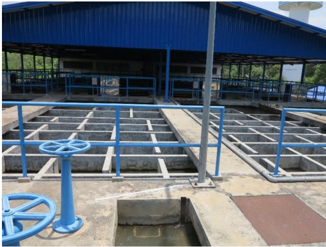
Roof at Sedimentation Tank
