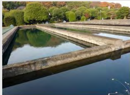
● Coagulation/sedimentation basin (rapid filtraion system)
