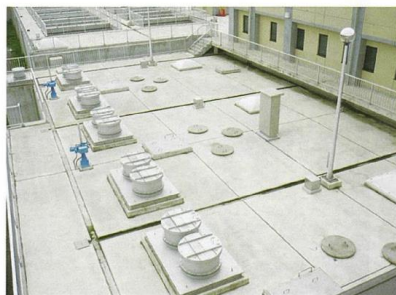
Activated carbon adsorption basin
