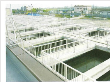
Activated carbon adsorption basin
