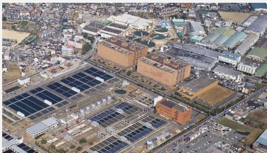
Figure 1 Murano Water Treatment Plant
