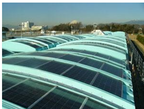
Solar power generation system on the rooftop of a water treatment plant
